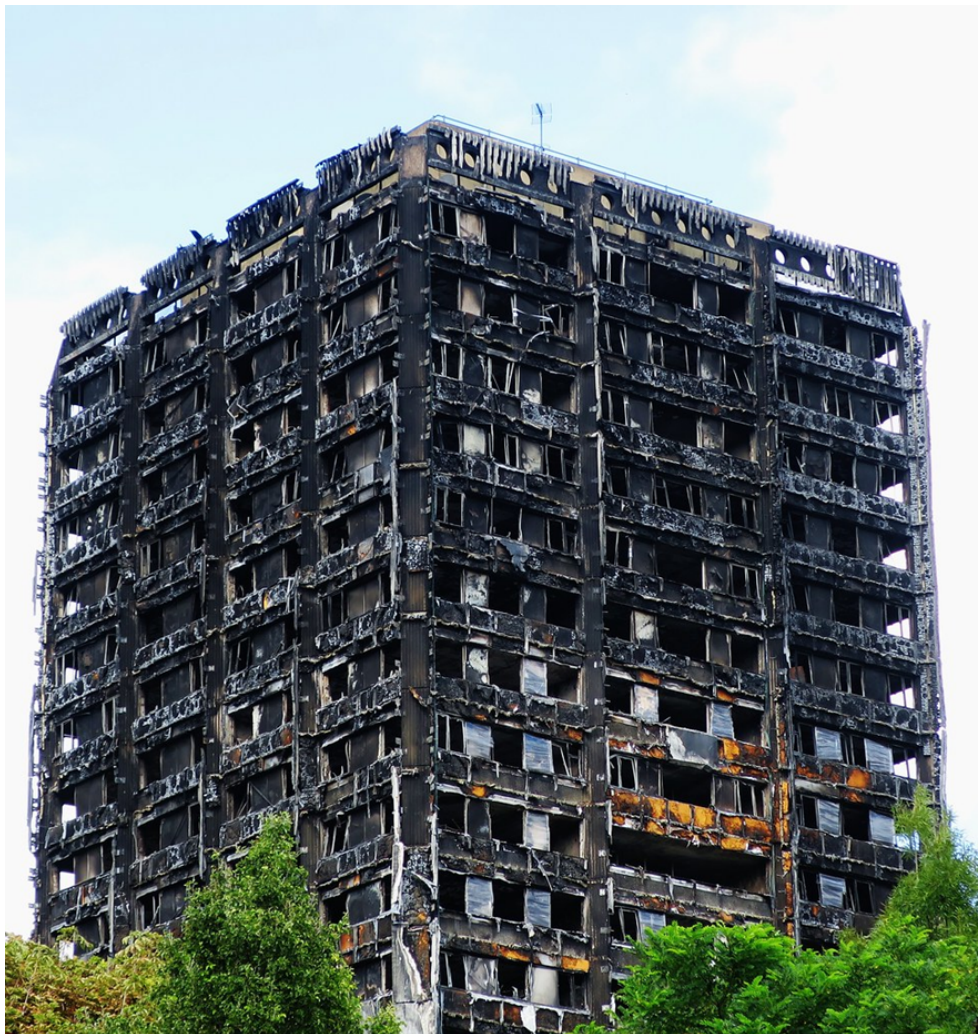
Figure 1.2: Grenfell Tower, London
