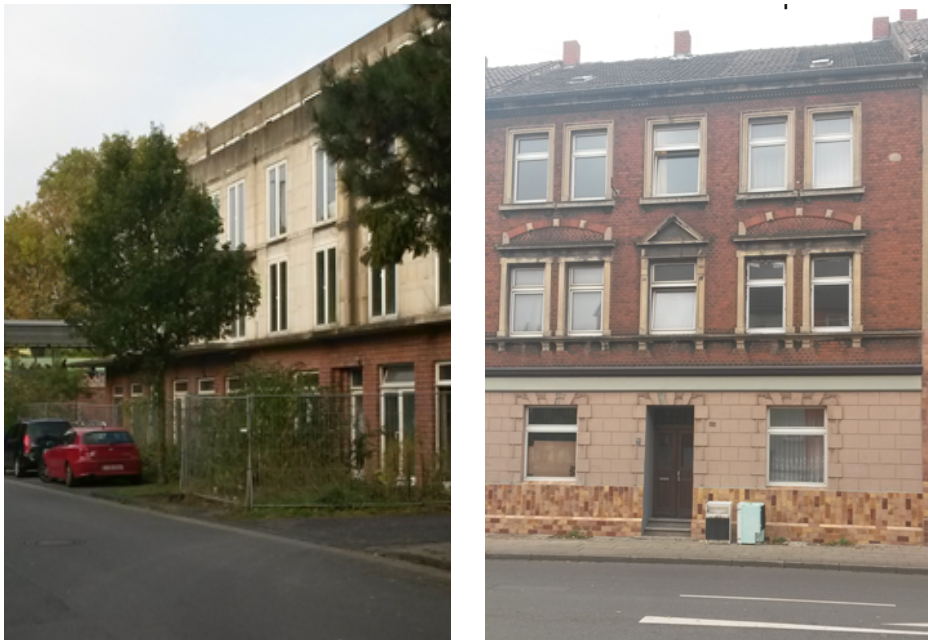
Figure 2.6: Under-maintained property rented out near Essen’s railway station (left), and another one in Old Essen (right).
