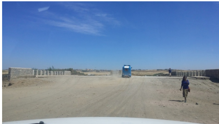
Figure 9: The new road to Dingur neighbourhood
